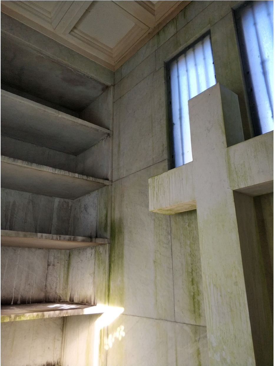
The interior of the Cheylesmore Mausoleum is panelled in white marble. The cross in the centre is the first memorial, around which the mausoleum was constructed.
